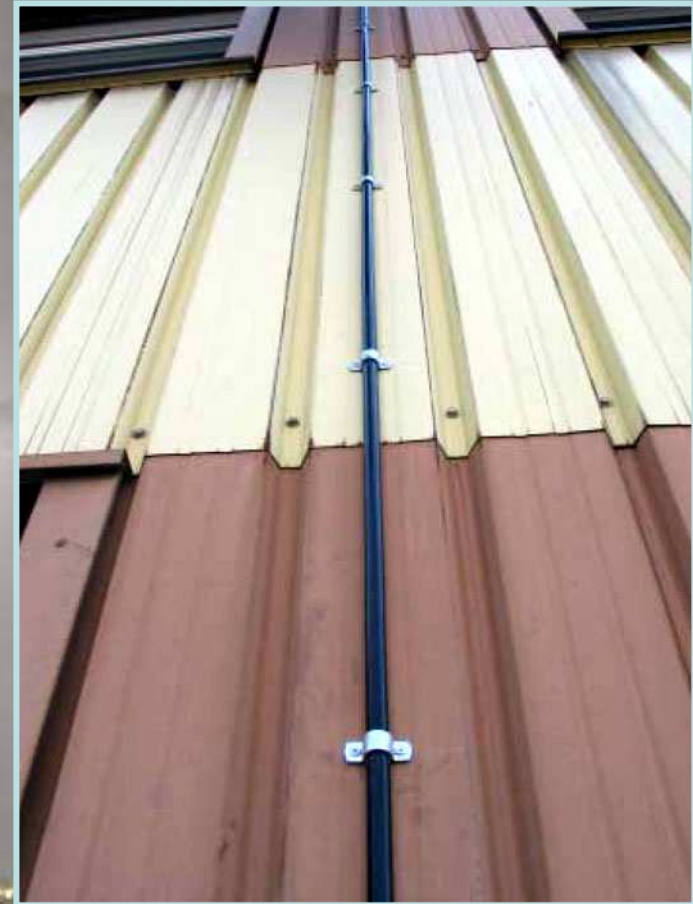
HVI ® installation on the facade
