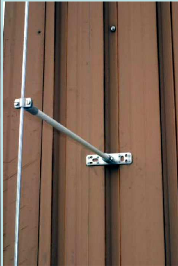
Installation of the distance holder
